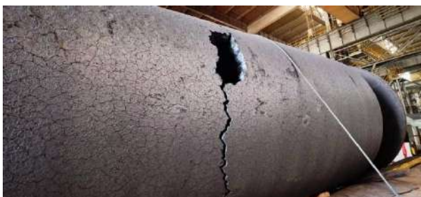
Full circumferential crack, coiler drum
